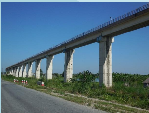
The high-rise approach bridge
