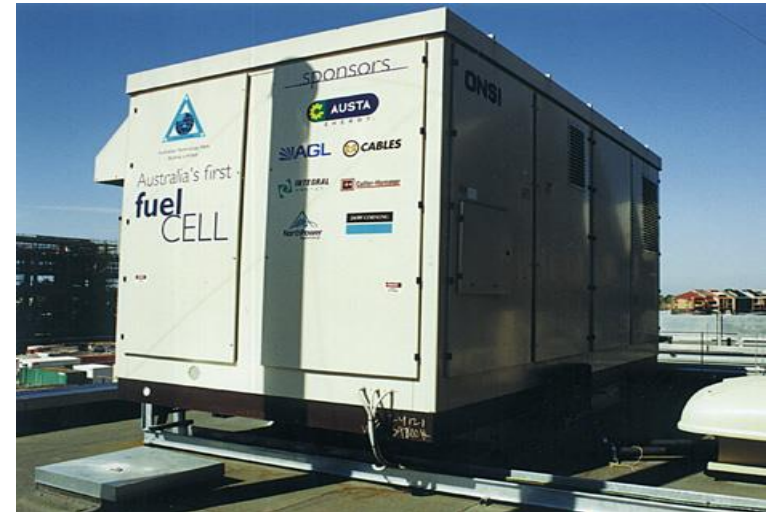
200-kW natural gas fuel cell plant in Sydney
