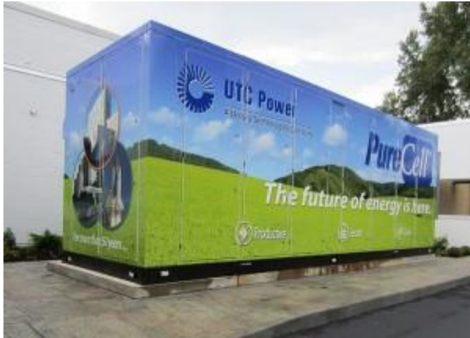
400-kW hydrogen fuel cell plant in Connecticut
