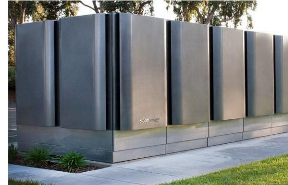
37-MW natural gas and biogas integrated fuel cell plant in California
