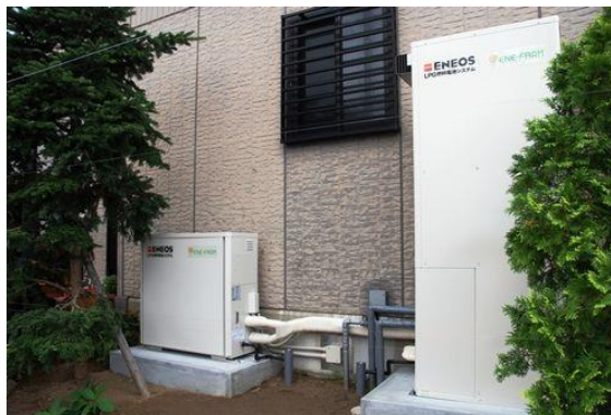
0.3 to 1-kW domestic hydrogen fuel cell in Fukuoka Prefecture
