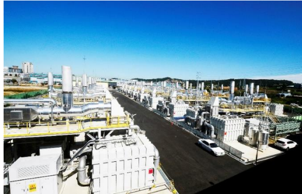
59-MW fuel cell park comprises 21 fuel cell power plants in Pyeongtaek
