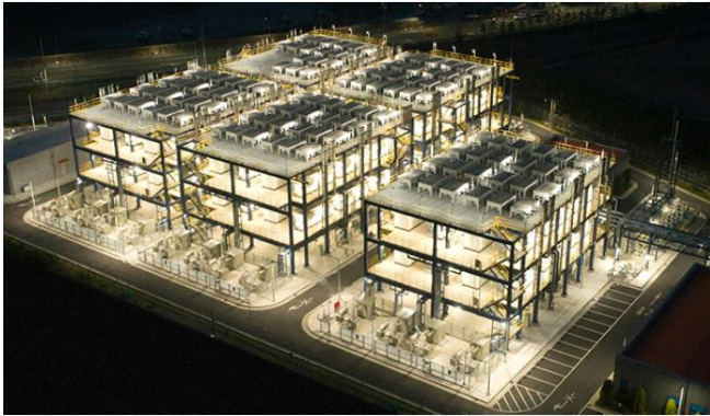
400,000-MWh year -1 hydrogen fuel cell plant in Seosan
