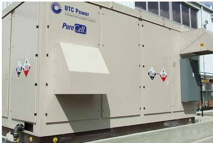
Natural gas fuel cell plant in New Jersey
